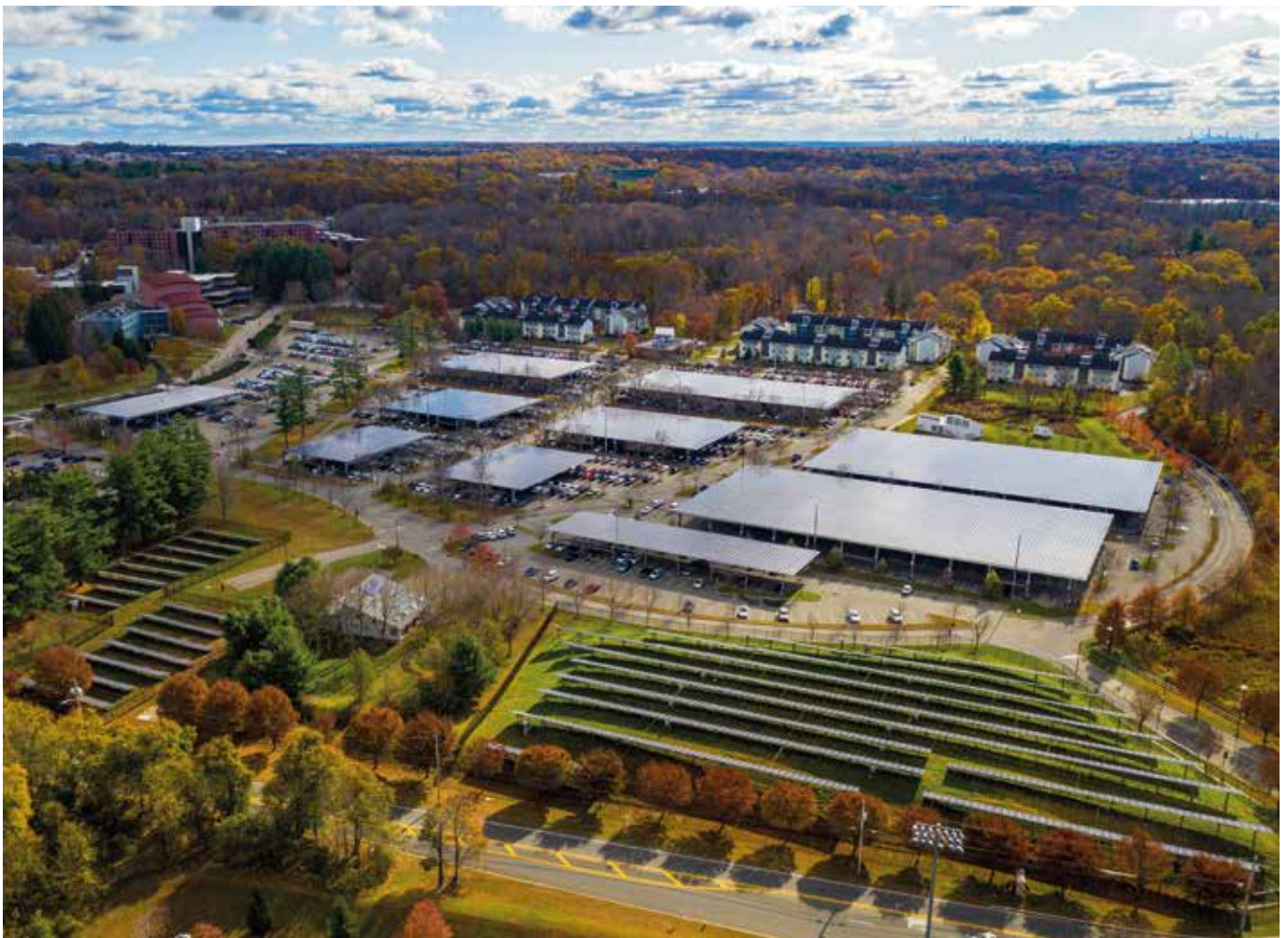
Vitol's rooftop and parking canopy system at Ramapo College, NJ, USA is capable of generating 5.1MW of solar energy.
